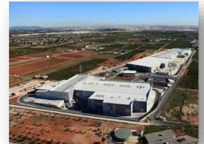
Composting plant (Asturias, Spain)
